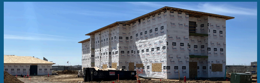
STRECK INC.: Units under construction in the Spring of 2022
